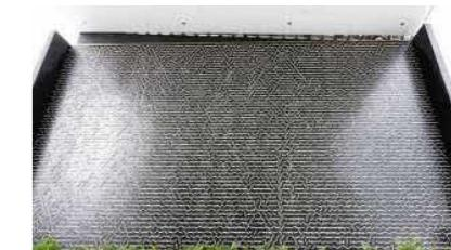
Comprising over 7,000 hinged metal channels that tilt as rainwater flows through, the striking Tipping Wall directs water to a catchment area below, where it is reused to sustain this mesmerising display of motion.
